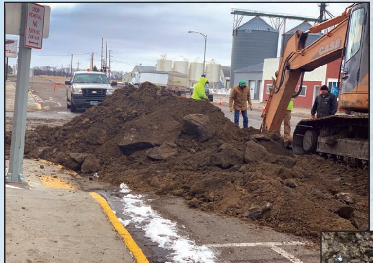
Limiting the excavation footprint on Highway 18 saved on repair expenses.
